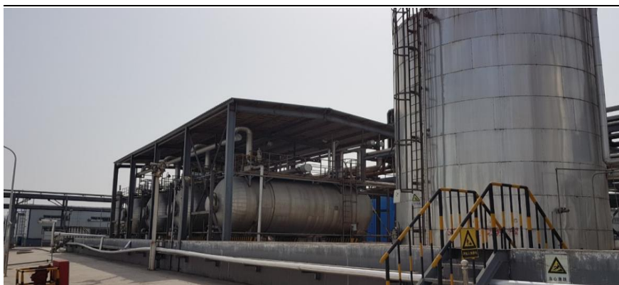
Figure 4: Processing storage tanks at the sodium hydrosulfite plant
