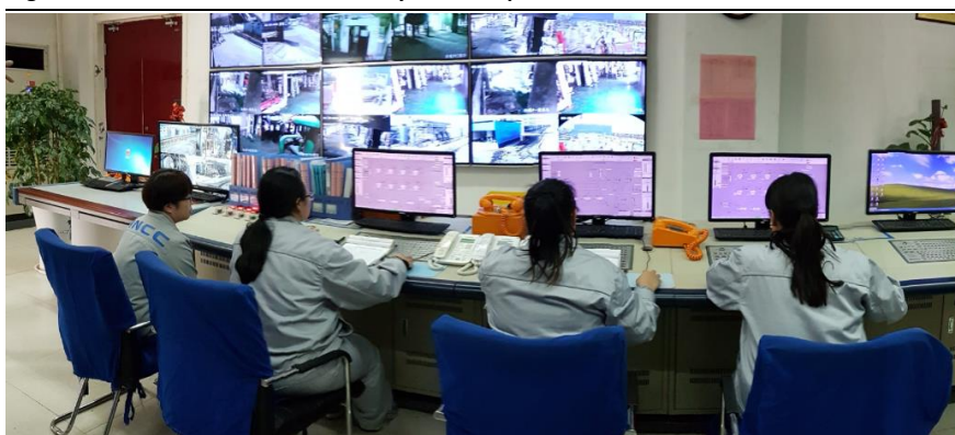
Figure 3: Control centre at the sodium hydrosulfite plant
